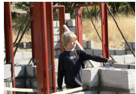
Jeremy offers help with grouting
